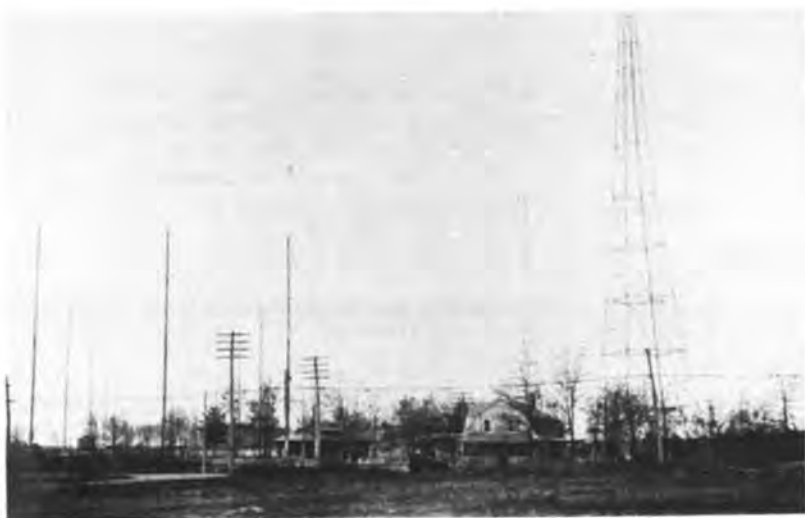
1924 - WIM/WCC TRANSMITTER SITE, RCA STATION AT MARION, MASSACHUSETTS.
